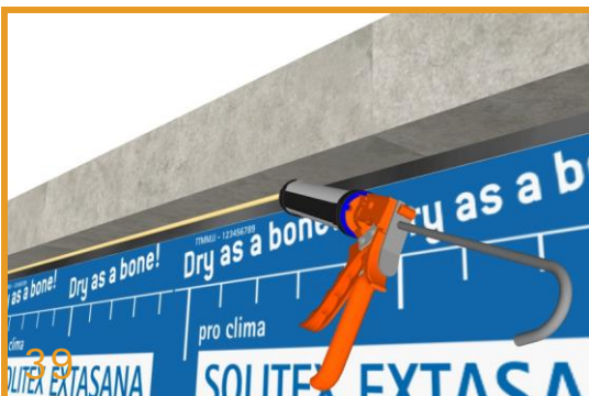
39 Seal to the Soffit Using ORCON® CLASSIC The SOLITEX EXTASANA® 30 mm overlap should be adhered to the soffit using a bead of ORCON® CLASSIC. (See matrix at step 61 for compatibility).
