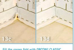
provides elasticity of the connection once dry to allow for building movement.
